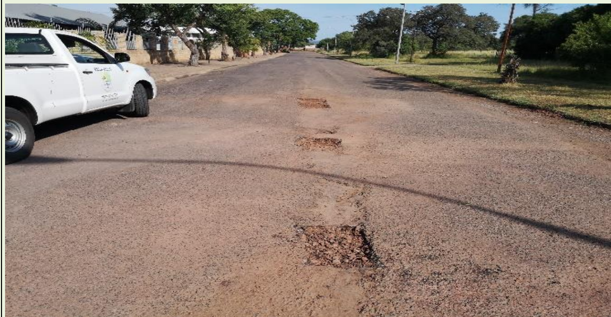
Damaged road with potholes
