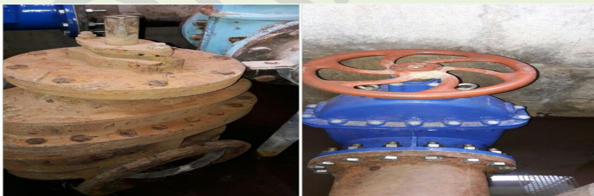
Replacement of old Valves at 7ML Reservoir
